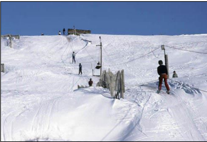
'Yad Moss 2000' rope tow circa 1983. Skiers used a car seatbelt and a metal hook to hold on to the heavy rope
