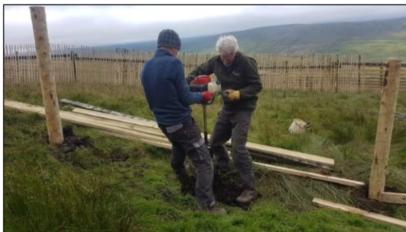
A petrol auger makes light(er) work of digging the post holes
