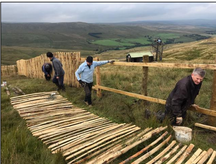
The new five-foot chestnut paling courtesy of Sport England should improve user management, snow capture and shelter in the queuing area
